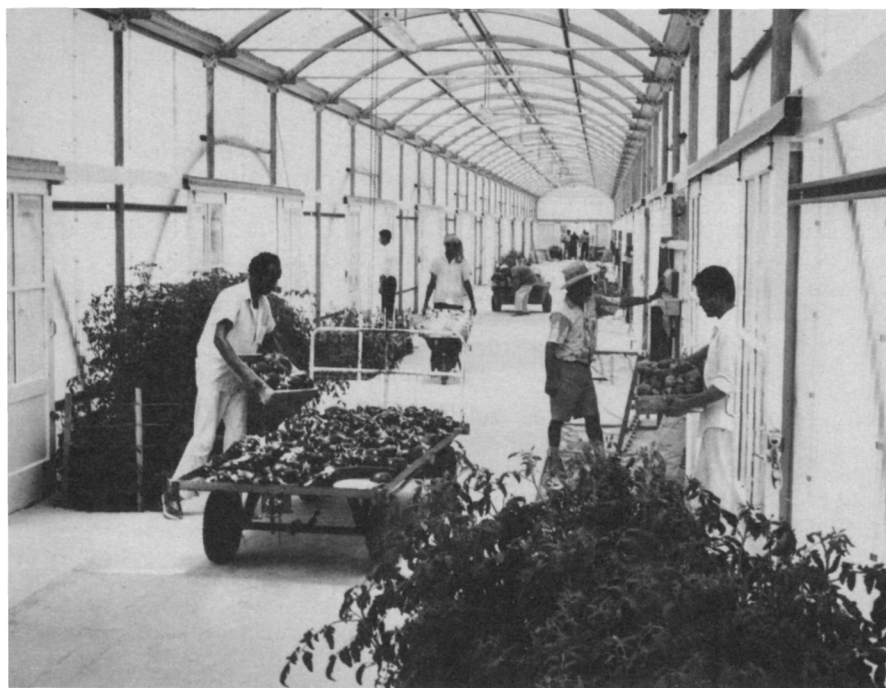
Fig. 1. Doors leading from central corridor into air-inflated greenhouse. Air is exhausted overhead.
