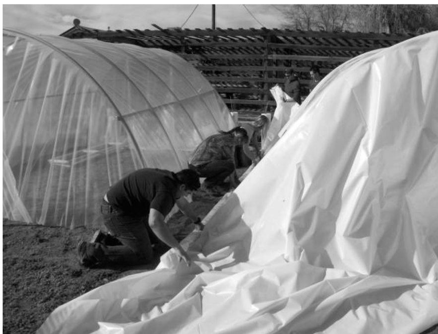
Fig. 1. Students and teaching assistants apply opaque polyethylene as glazing on one of five 12 \times 15 -ft ( 3.7 \times 4.6 m) hoop houses as part of the laboratory sections of the Introductory Plant Science (HORT/AGRO 100G) class at New Mexico State University at Las Cruces in Spring 2013. Clear polyethylene can be seen on the hoop house to the left.
