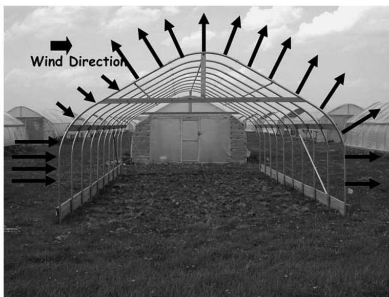
Fig. 2. High tunnel structure indicating the wind loading (inward as positive pressure, and outward as negative pressure) for the wind direction as shown (Center for Plasticulture, 2008).
