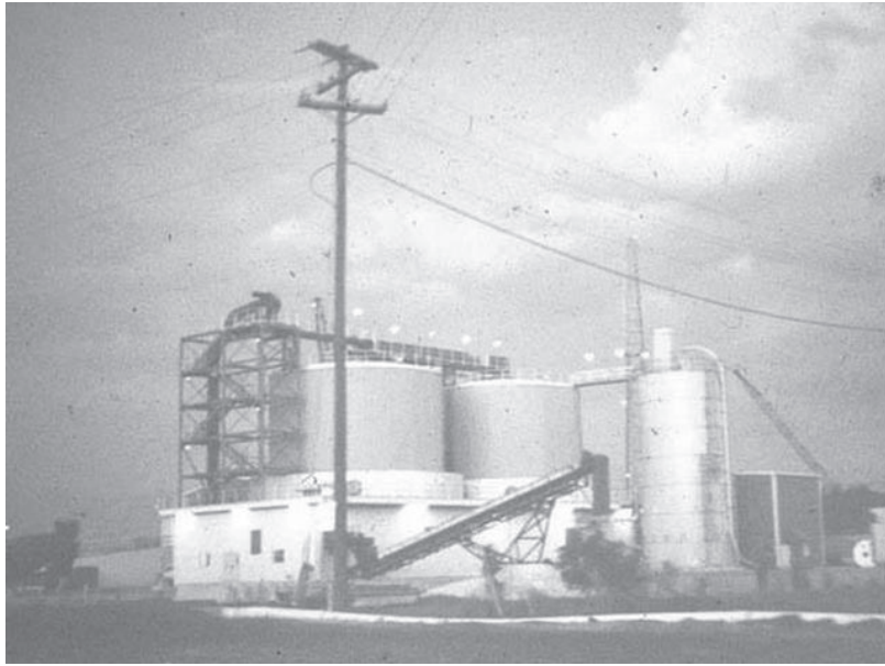
Fig. 4. Silo type composting system, Lake Buena Vista, Fla. Photo by G.E. Fitzpatrick.
