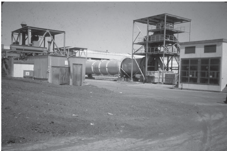
Fig. 2. Rotary drum composting system, Al Ain, United Arab Emirates. Photo by G.E. Fitzpatrick.
