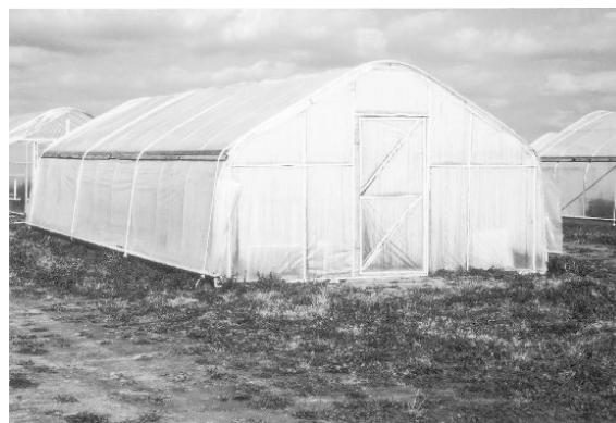
Fig. 1. High tunnel constructed using the New Hampshire design developed by Otho Wells, University of New Hampshire.
