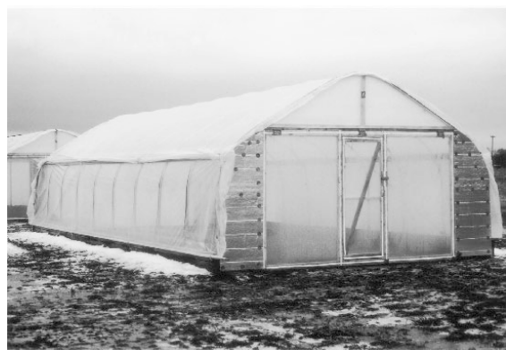
Fig. 2. High tunnel constructed using the Penn State design developed by researchers and extension specialists at the Penn State High Tunnel Research and Education Facility.
