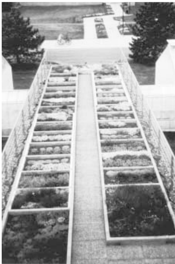
Fig 1. Sopranature green roofing system installed in November 1994 on a one story existing building at Université Laval, Québec. The 12 experimental plots on each side of the walkway form six experimental units. Each experimental unit consists of two plots of the same depth, 2, 4, or 6 inches (5, 10, or 15 cm), placed side by side.
